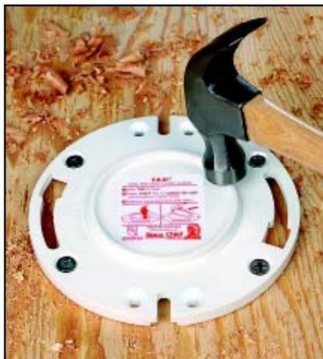
Hit the raised rim of the TKO until the knockout cracks loose.
