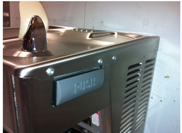
Fasten Basin Assembly in place.
