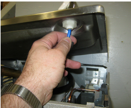
Remove Bubbler Water Line
