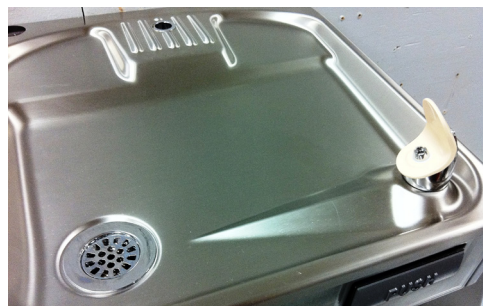
Exchange Bubbler hardware.
