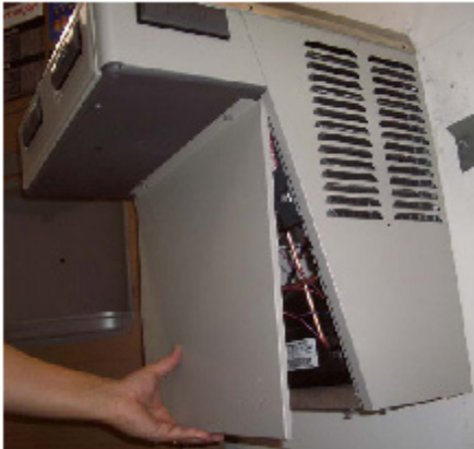
Remove Front Panel
