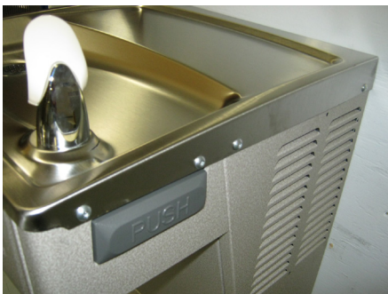
Remove Basin Fasteners
