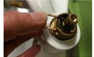
18. Slide the copper clip back into the valve body on top of the cartridge. If you have trouble installing this, please refer to the special note at the end of this document.
