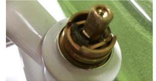
19. Slide the double-D washer onto the brass cartridge stem.
