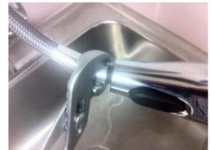
7. Hand-tighten the hose to the wand. Then, using the pliers on the hose collar, turn 1/8 of a turn.
