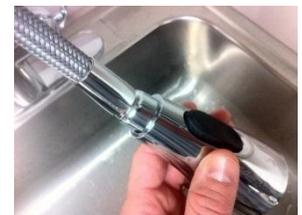
9. Remove the towel or bag from the hose and set the wand into the receptor.
