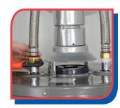
or pipe wrenches. If the piping was soldered into place, use a tubing cutter to cut the pipe.
