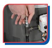
connect them. Assemble and tighten each fitting with two pipe wrenches. Install the union fitting last because it connects the new line to the existing line. When finished, open the gas supply valve. Test for leaks by applying a wet, soapy sponge to the new gas fittings. Check for bubbles. If there is a leak, bubbles will form on the surface and you will have to refit the joint.
