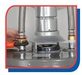
or at the flare fitting if the gas supply line is copper. Disconnect the water lines above the tank using two adjustable wrenches or pipe wrenches. If the piping was soldered into place, use a hacksaw or tubing cutter to cut the pipe. Make sure the cuts are straight.
