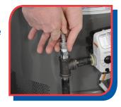
connect them. Assemble and tighten each fitting with two pipe wrenches. Install the union fitting last because it connects the new line to the existing line. When finished, open the gas supply valve and turn the water on. **Turn on the water at the tank, then turn on one or more hot water faucets to bleed air out of the system.**
