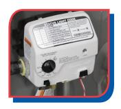
once every 10 seconds until pilot is lit. Continue to hold the thermostat knob down until the LED "STATUS" light begins to blink. Release the knob and rotate it to the desired temperature setting. Set the control at a temperature between 118 and 123 degrees.
