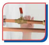
check for bubbles. Test all connections. If there is a leak, bubbles will form on the surface and you will have to refit the joint. Inspect water lines for leaks.
