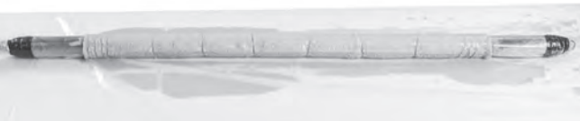
Figure 32 – Patch Properly Wet Out And Secured With Doubled Over Elastic Bands
