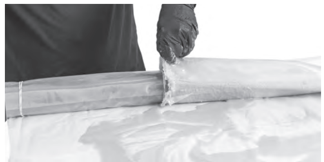
Figure 29 – Inserting The Packer In Patch
