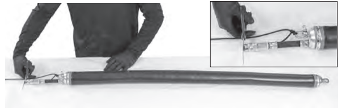
Figure 23 – Cutting Containment Tube To Length For Full Packer
