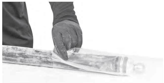
Figure 12 – Inserting Packer Into Sleeve
