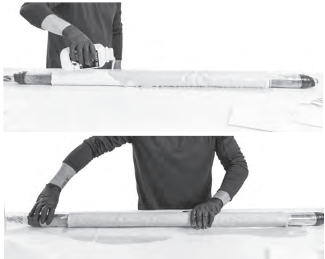
Figure 33 – Wetting Out The Patch On The Packer
