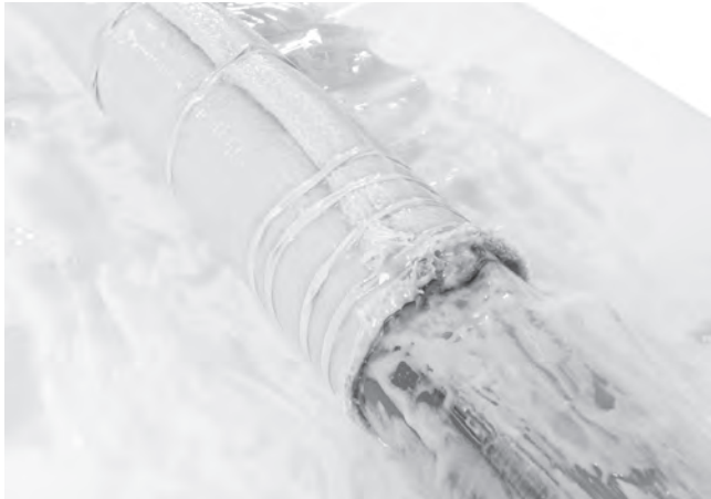
Figure 30 – Gathering And Folding The Patch
