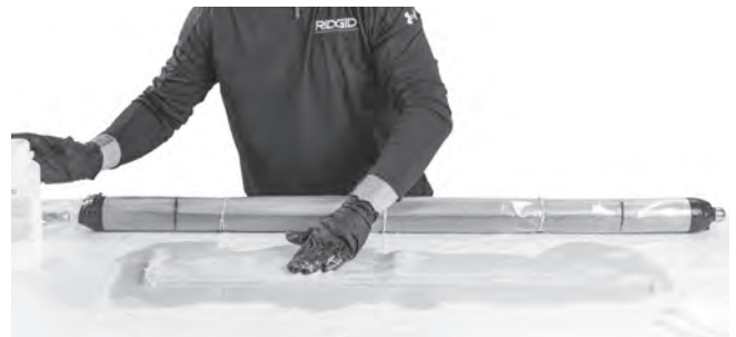
Figure 28 – Wetting Out The Patch Off The Packer
