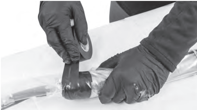
Figure 17 – Securing The Sleeve With Tape At The Back Of The Packer
