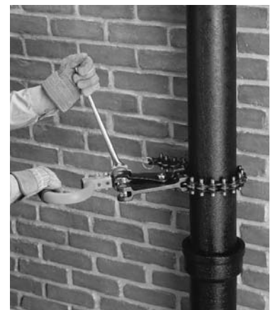
Cutting pipe in close quarters
